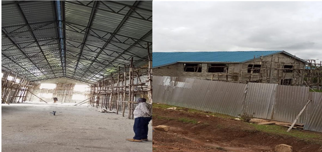
Figure 3 Inspection of On-going project (West Pokot County Milk Processing Plant- Kabichbich)
