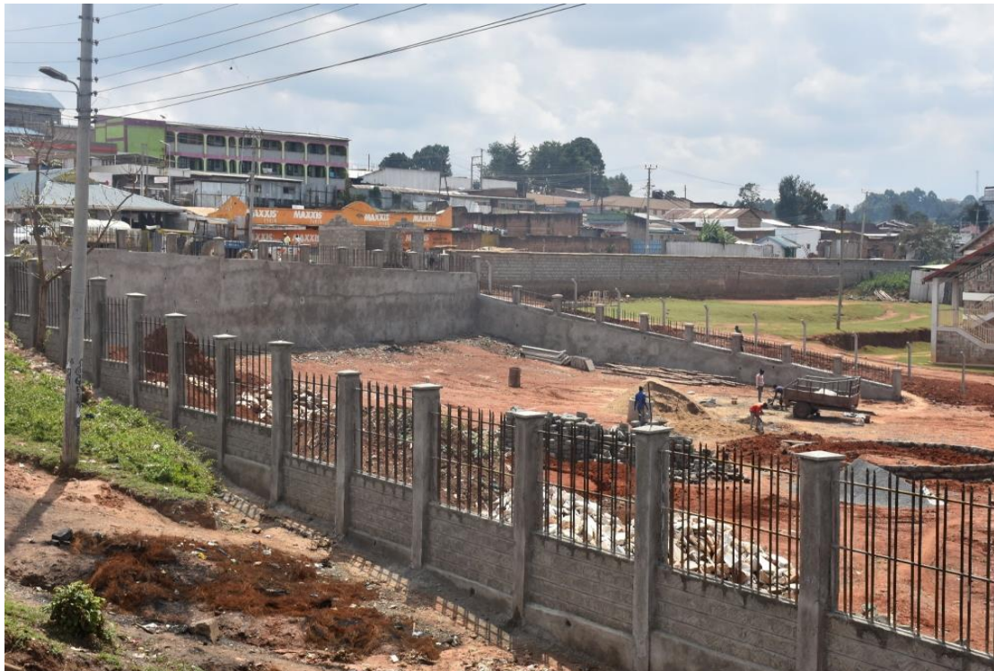
Figure 4: construction of recreational park at Makutano
