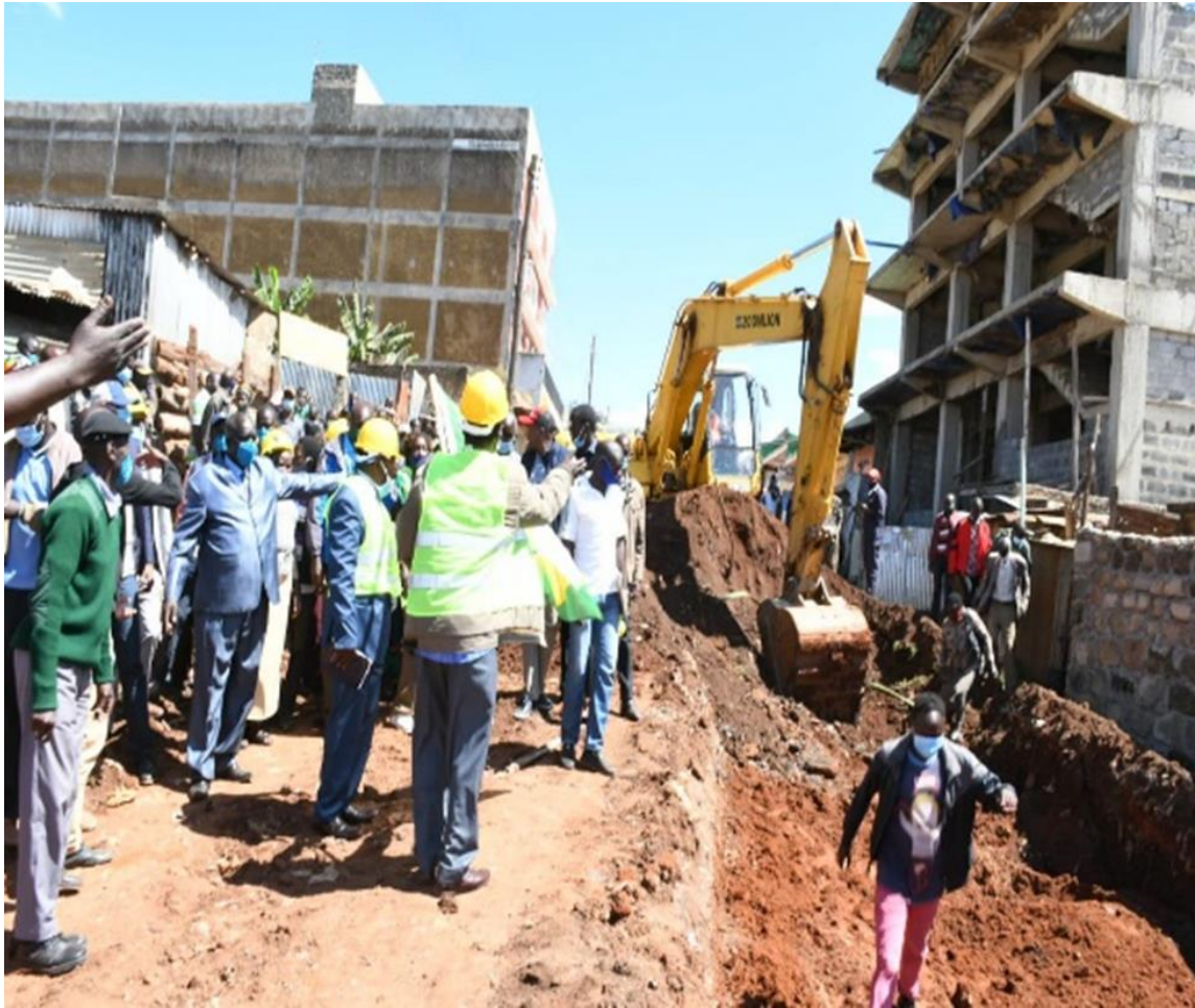
Figure 4: His Excellency the Governor launching tarmac works at Makutano town
