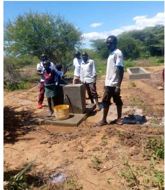
Tulungwo-Katukuri Water Supply
