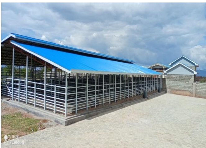
Nasukuta newly completed livestock holding pens
