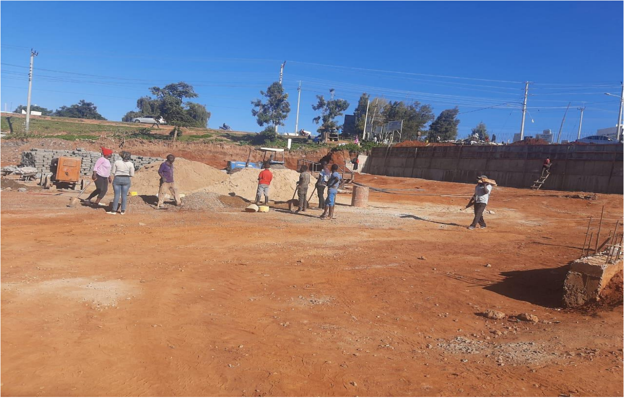
Figure Longoing construction of recreational park at Makutano town
