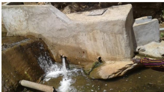
Orwa Irrigation Intake (left) and Kaminia Irrigation Civil works in progress
