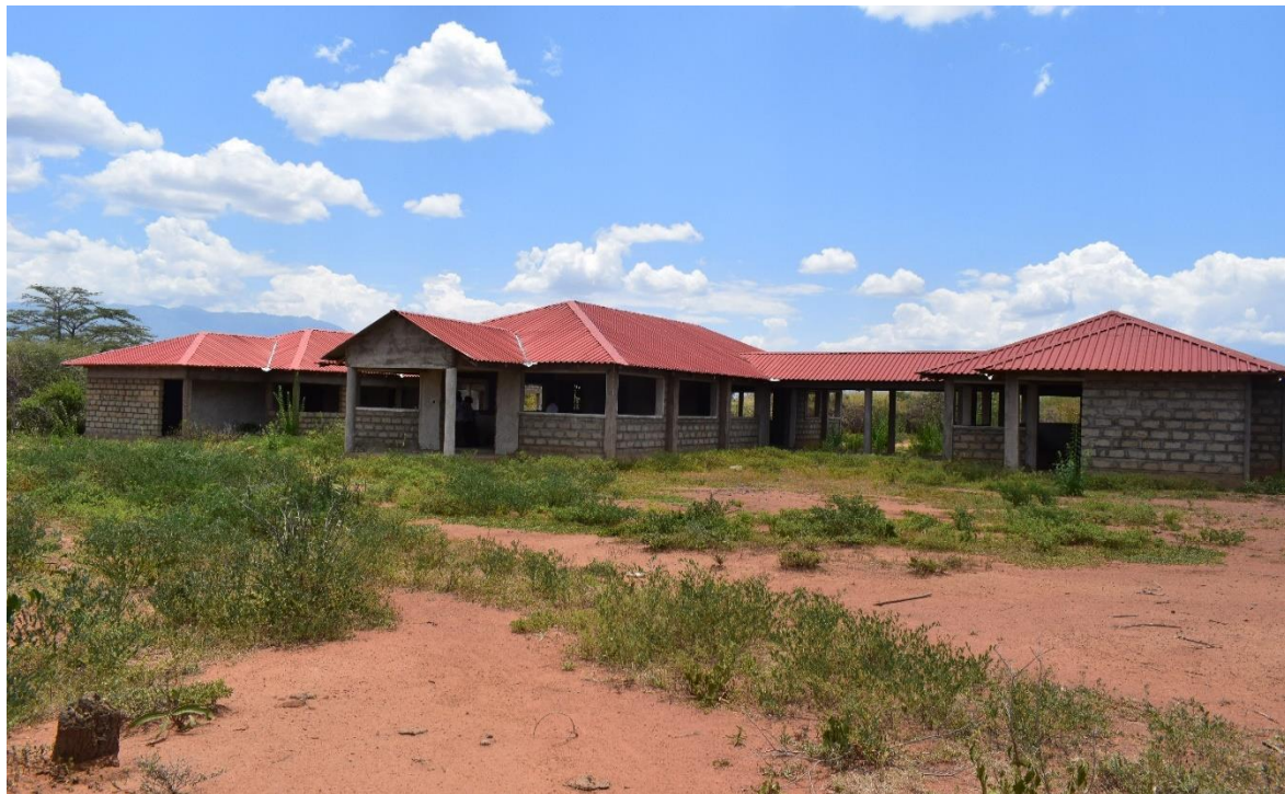
Figure 3 DISPENSARY FROM THE BACK SIDE
