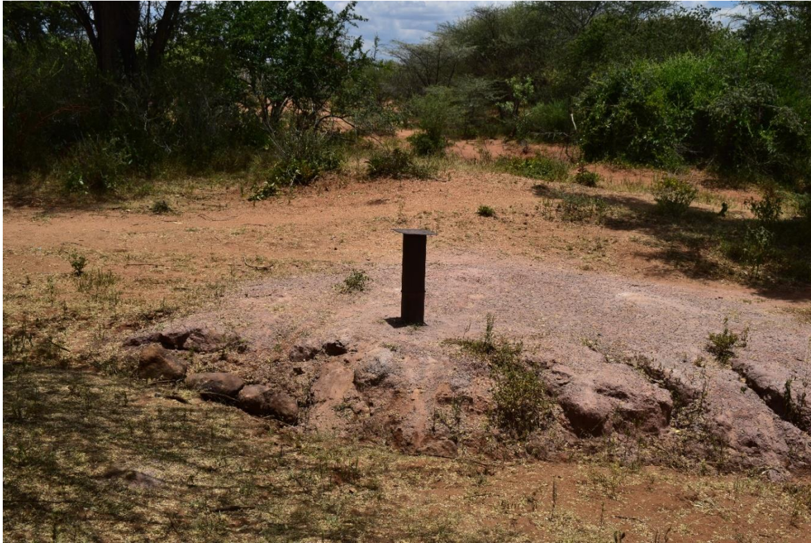
Figure 5 BOREHOLE DRILLED BUT NOT YET EQUIPPED
