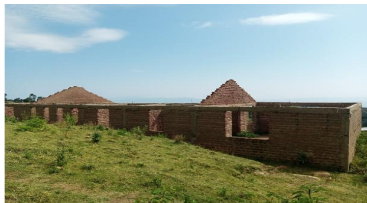
1. Ksera maternity construction at lintel level
