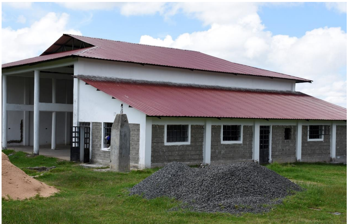
Figure 1 ongoing modern fire station at 90%
