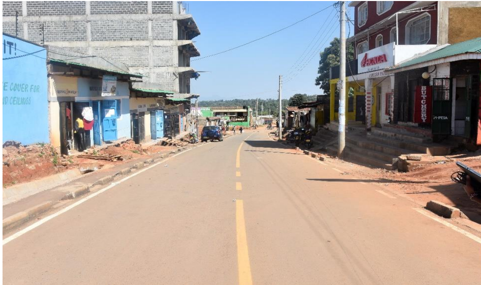
Figure 2 complete tarmac road at Makutano town under KUSP funding
