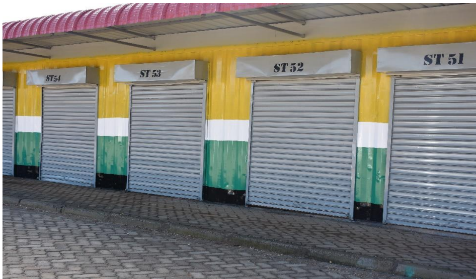
Figure 3 Complete paved market stalls at Makutano town
