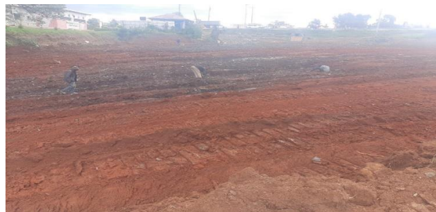
Figure 1 ongoing leveling of the recreational park at Makutano town
