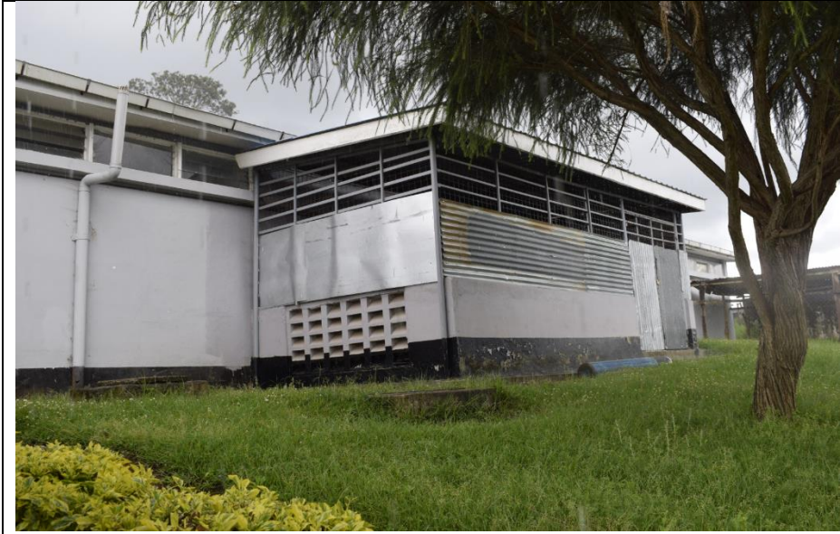
Oxygen Plant Housing Structure
