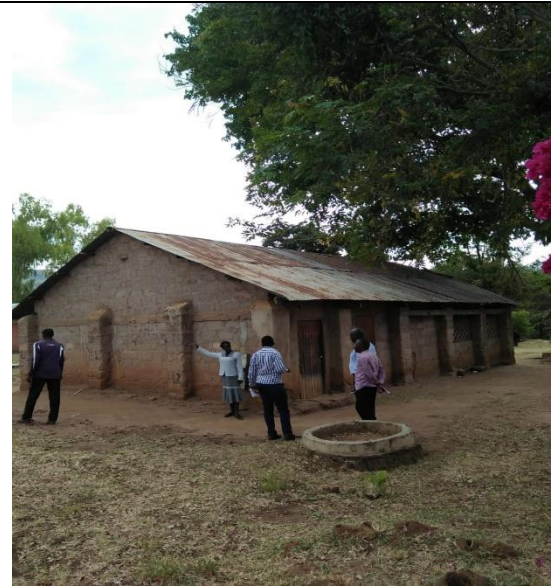
Figure3: Chepareria VTC workshop(C&J) Before renovation
