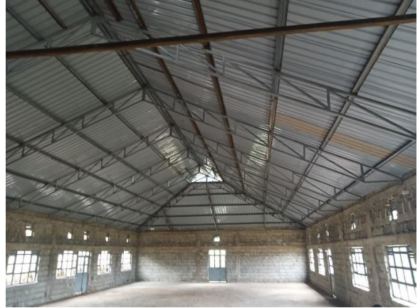
Figure 11: Roofing of multipurpose hall
