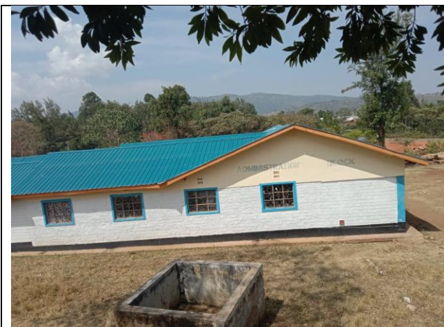
Figure 17: Rehabilitation of male and female hostel at Chepareria VTC
