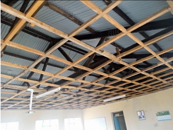
Figure 25: Twin workshop (which needs ceiling and wiring)
