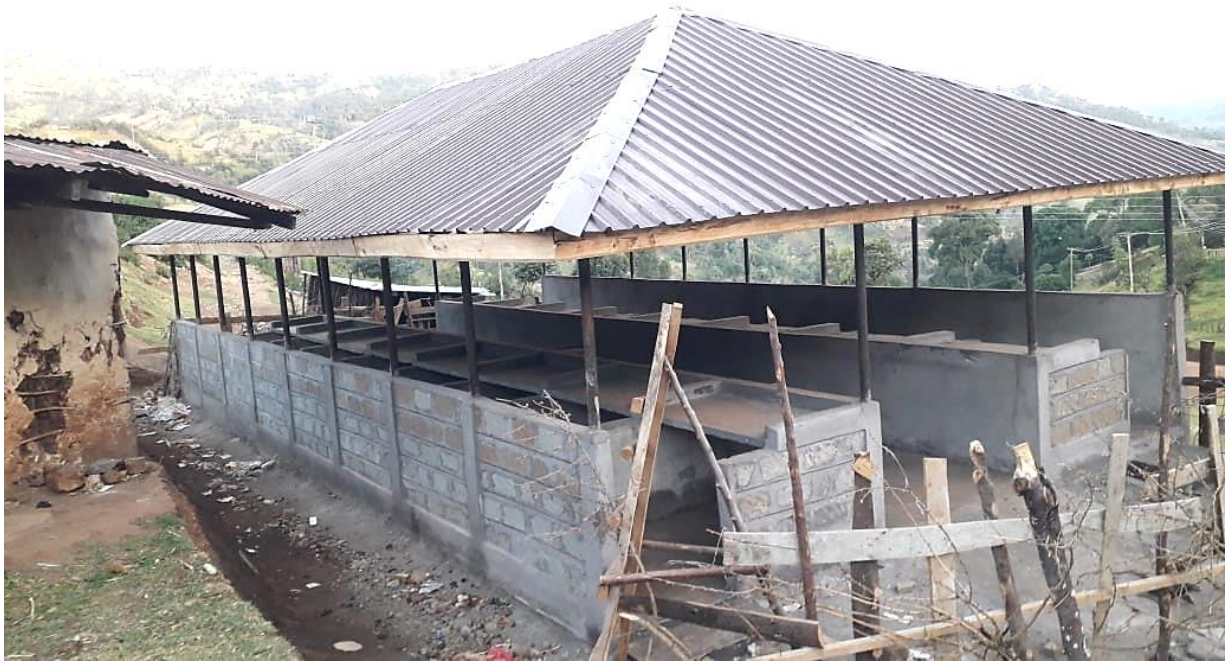
Figure 37: Sina Fresh Produce Market – Work in Progress
