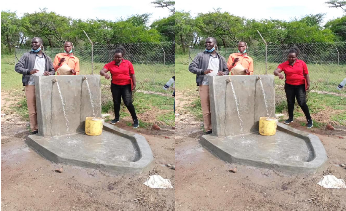
Figure 30: Upgraded Lokitonyala Borehole
