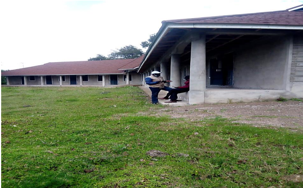
Figure 42: Ongoing Construction of Mtelo Conference Facility.
