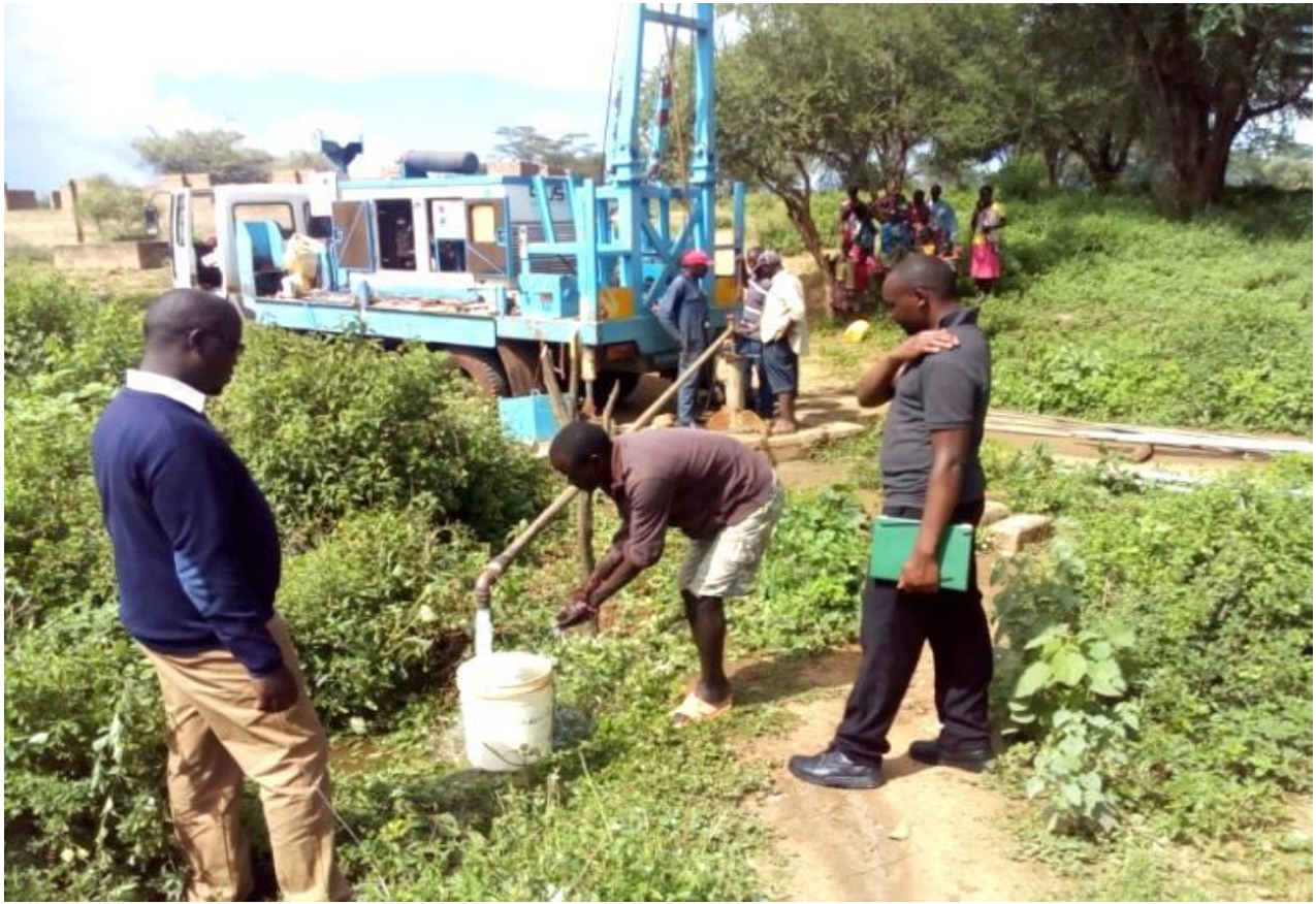
Figure 13: Pumping testing at Akiriamet borehole
