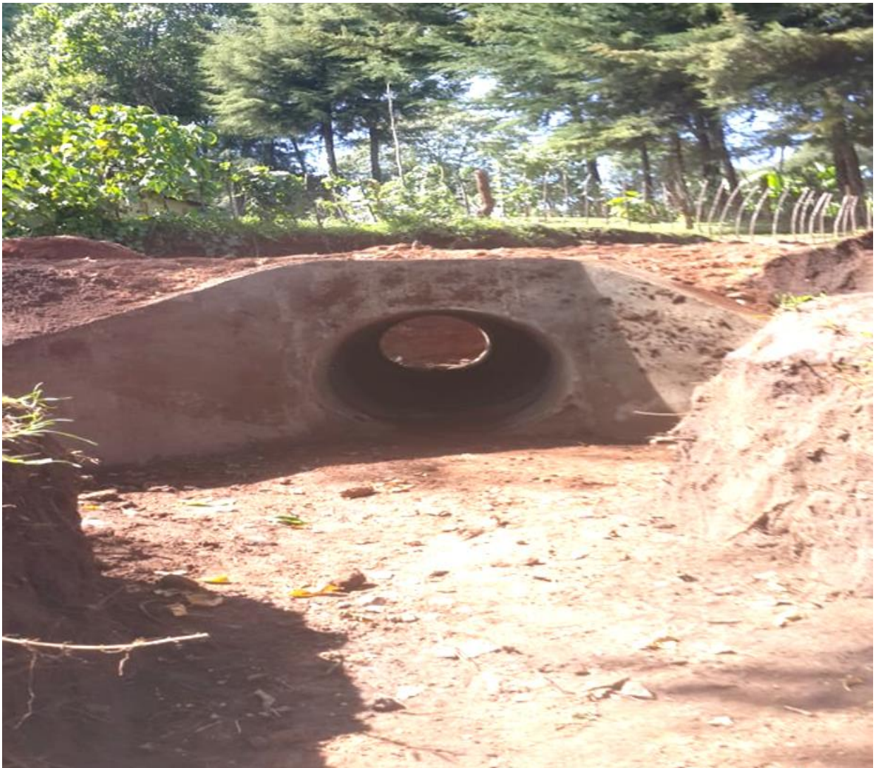
Figure 2: Culvert installation at Kapsurum, Siyoi ward.
