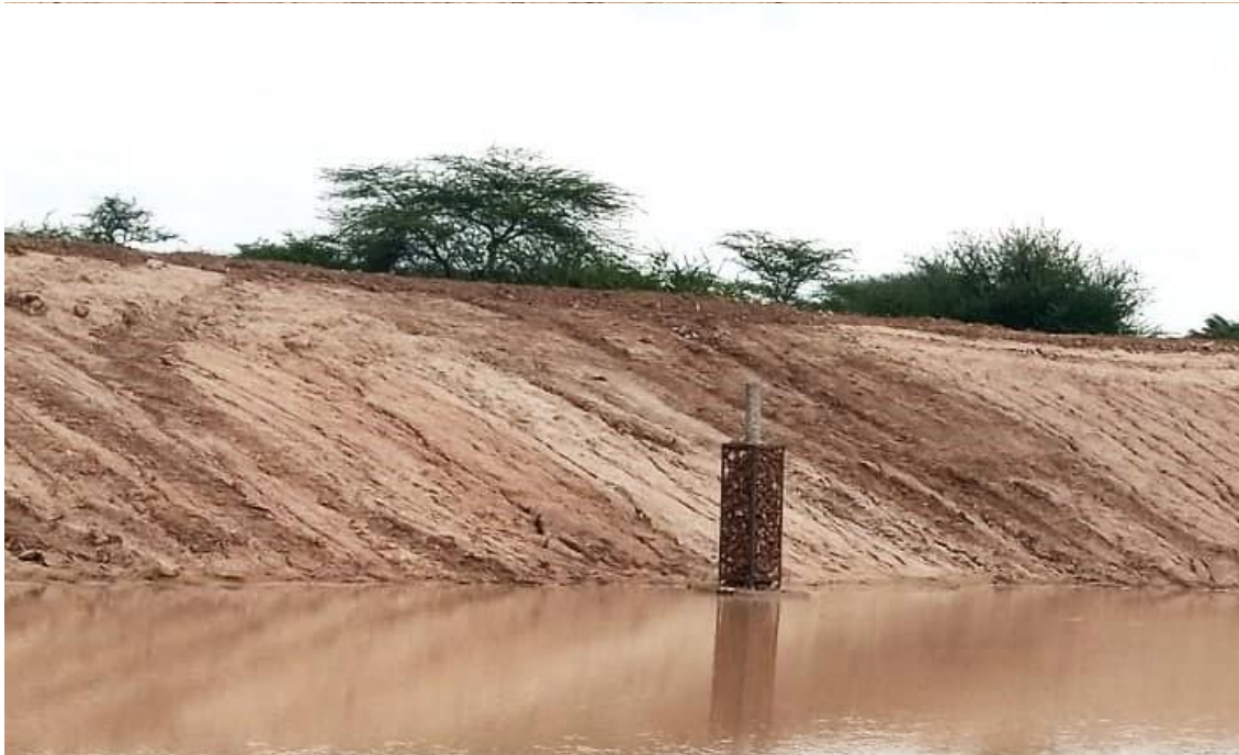
Figure 14: Newly Constructed Namoru Water Pan in Kodich Ward
