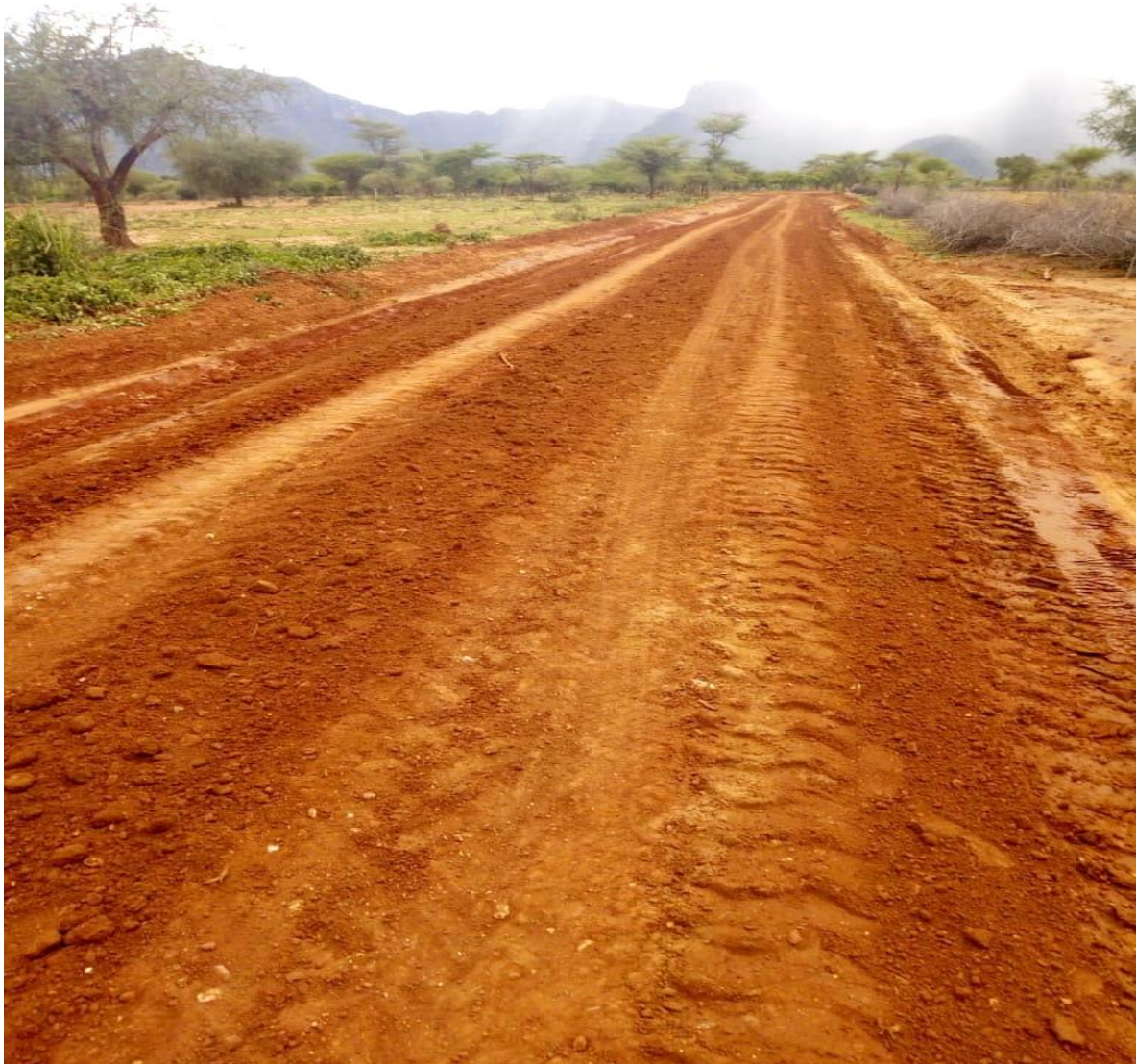
Figure 2: Kacheliba-Nakwapuo-Cherangan road grading
