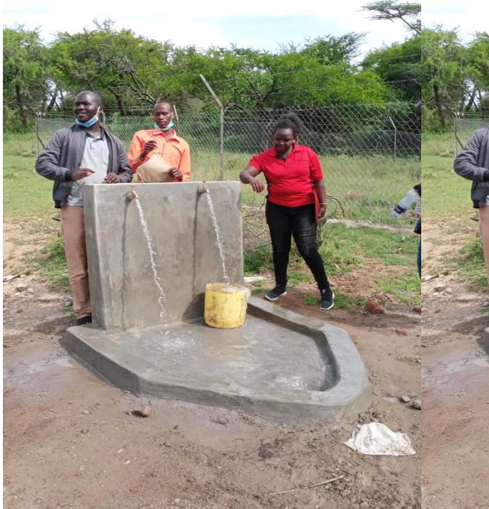
Figure 16: Newly Upgraded Lokitonyala Borehole
