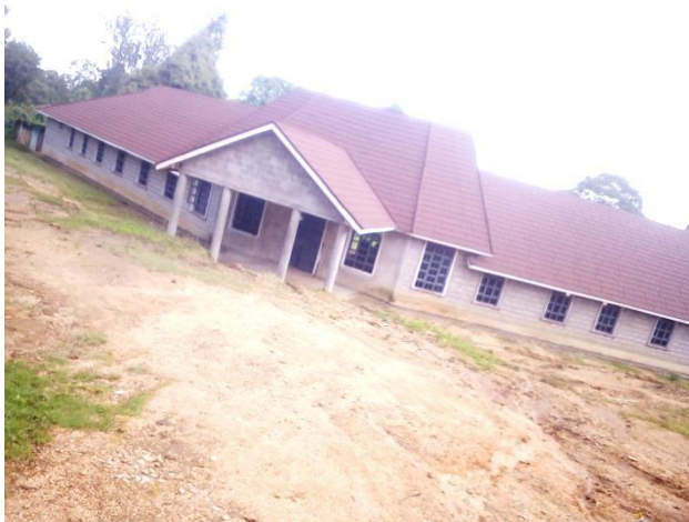
Figure 20: On-going construction of Mtelo cottages
