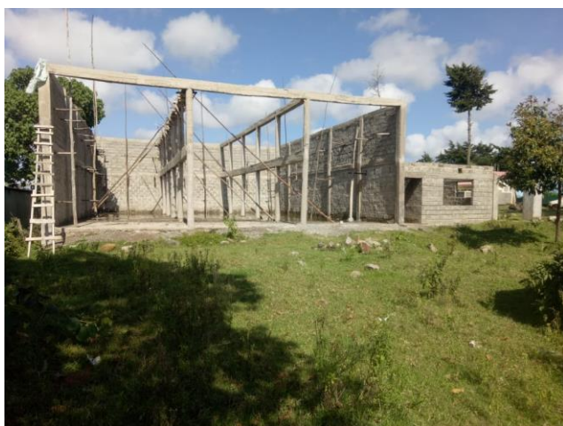
Figure 13: On-going construction of modern fire station at Kapenguria Municipality
