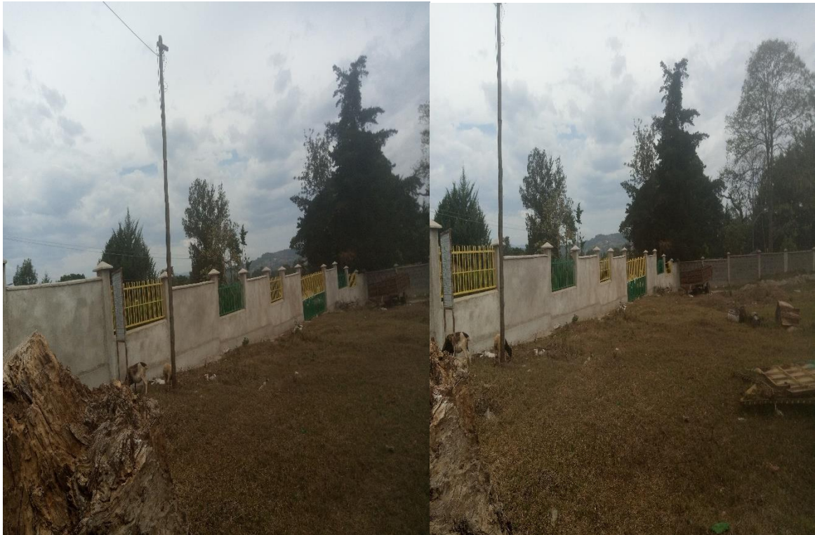
Complete Peremeter wall at Land Office
