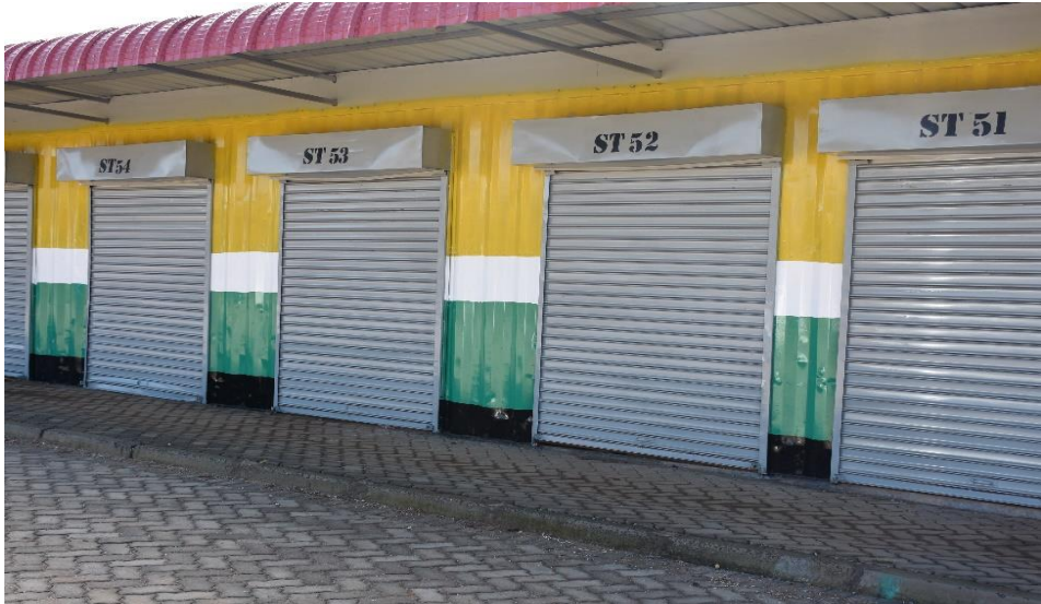
Complete paved market stalls at Makutano town
