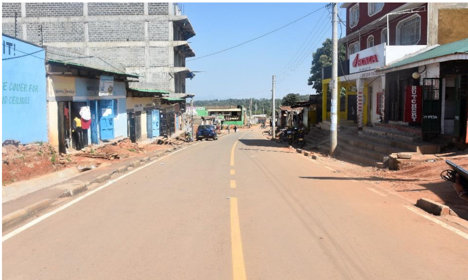
Tarmac road at Makutano town
