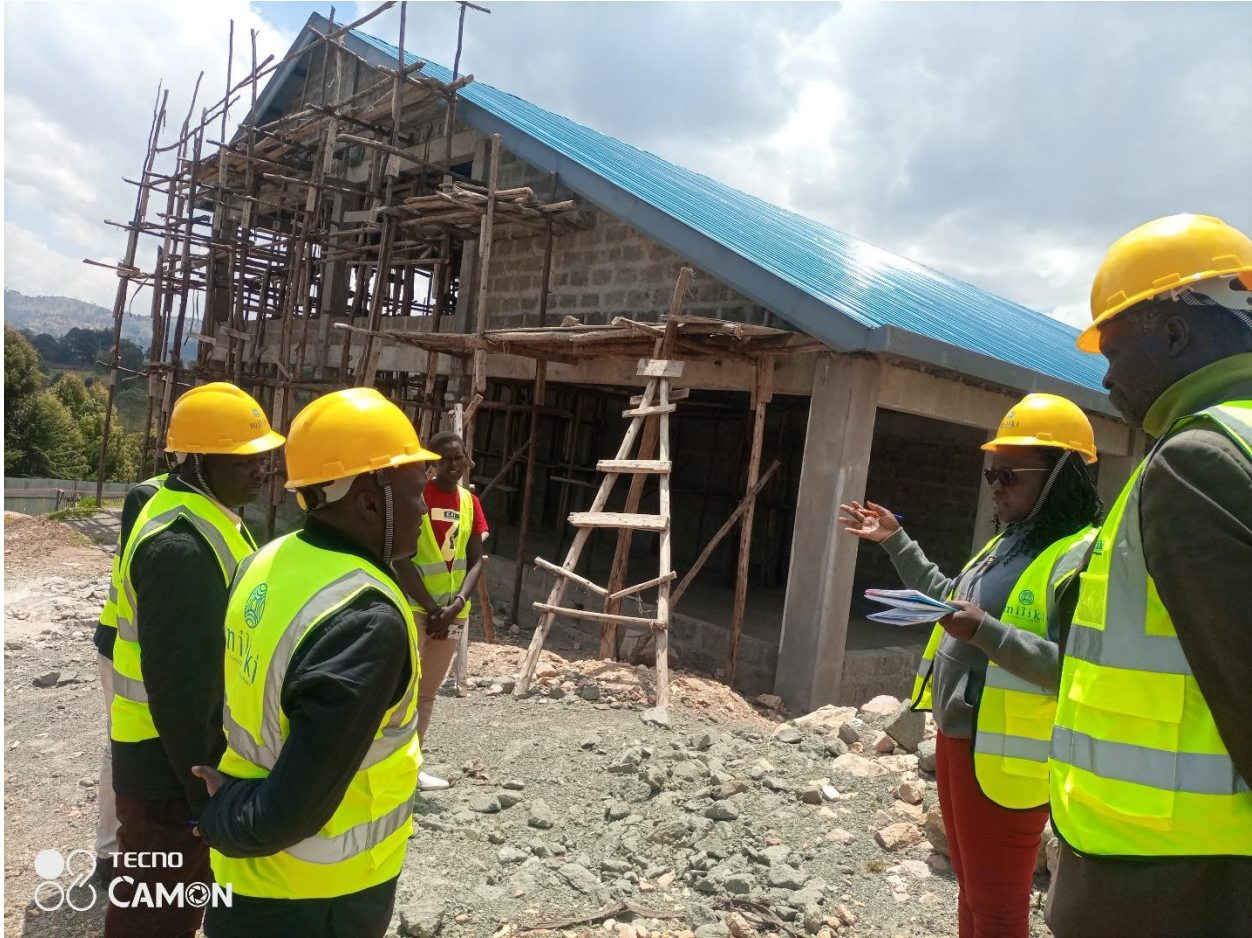
Figure 4 Construction of milk processing plant at Kabichbich
