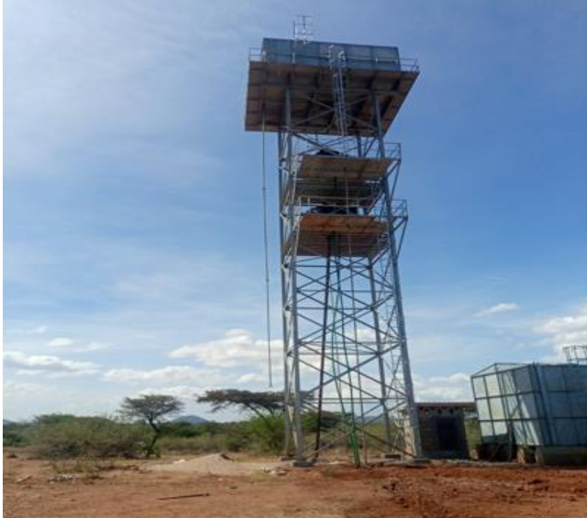
Figure 1 Elevated water tanks at Nasukuta Abattoir
